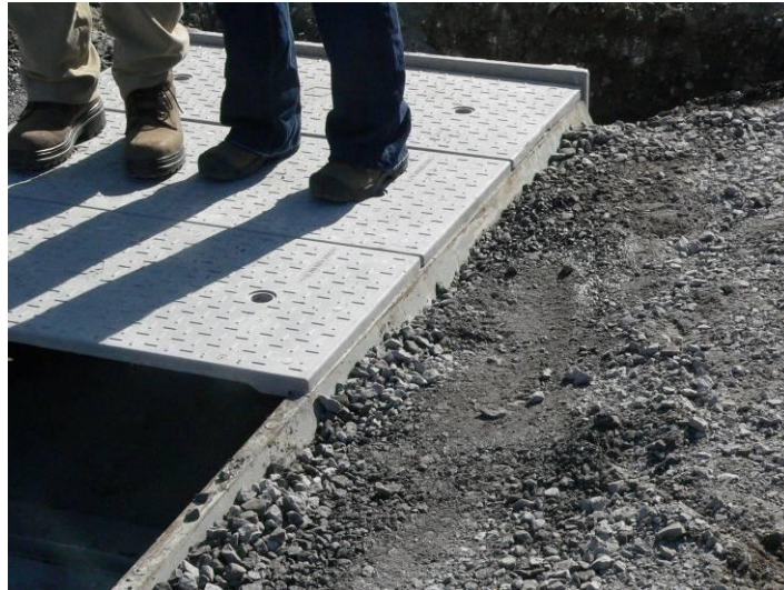
Figure 7 : Final level of the trench after installation
