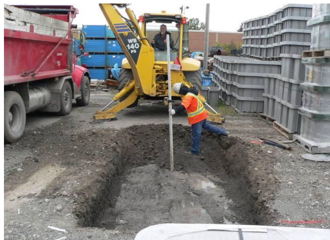
Figure 2 : Measure of the depth and width of the ditch.
