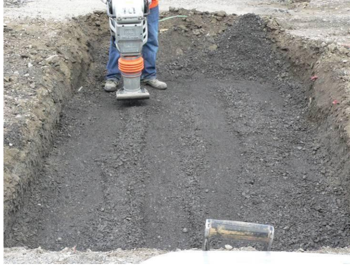
Figure 3 : Filling and compacting.
