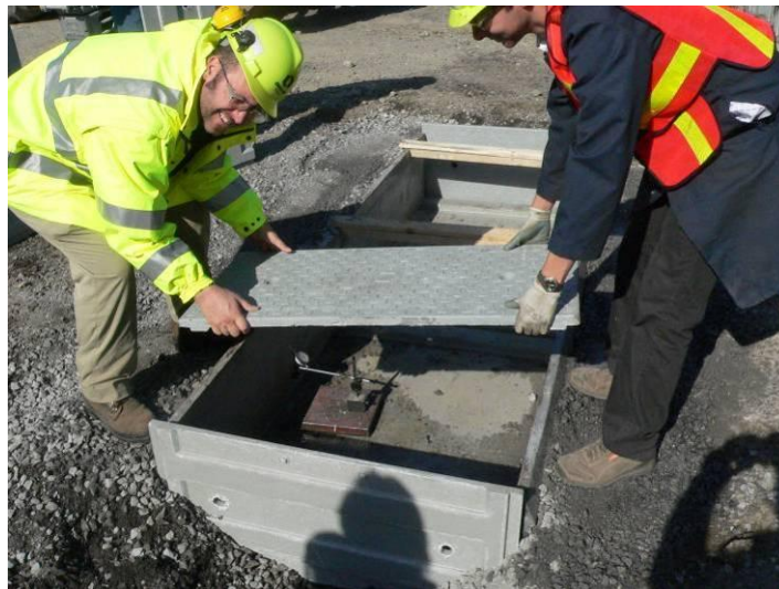
Figure 8 : Installation of the covers
