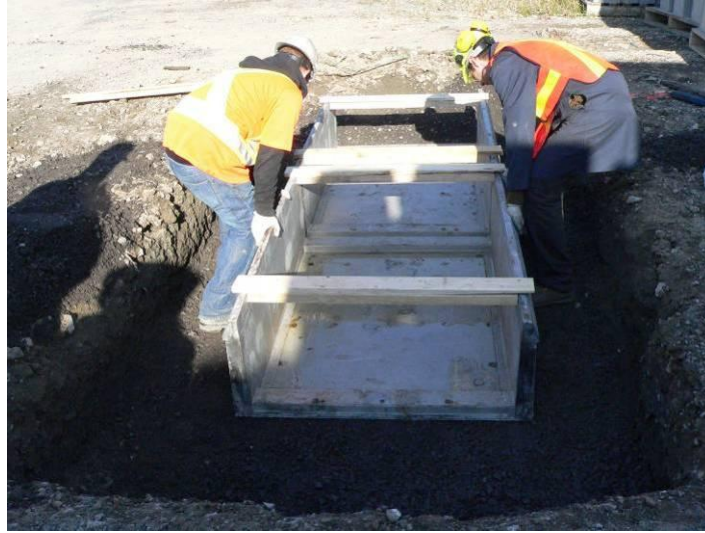
Figure 5 : Keep the wood blocks
