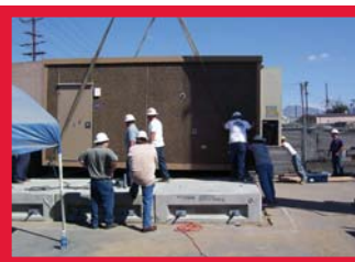
Set, anchor, and ground shelter and monopole.
