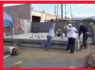
Work begins at 8:00 AM, with the last block set by 9:00 AM.
