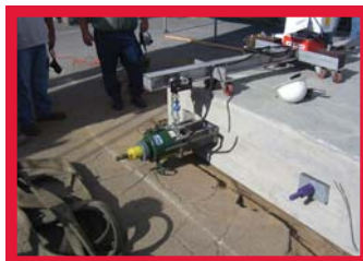
Post-tensioning to 100%, foundation complete by 10:30 AM.
