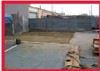
Previously prepared site.
