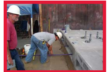
Install post-tensioning hardware and post-tension to 50%.
